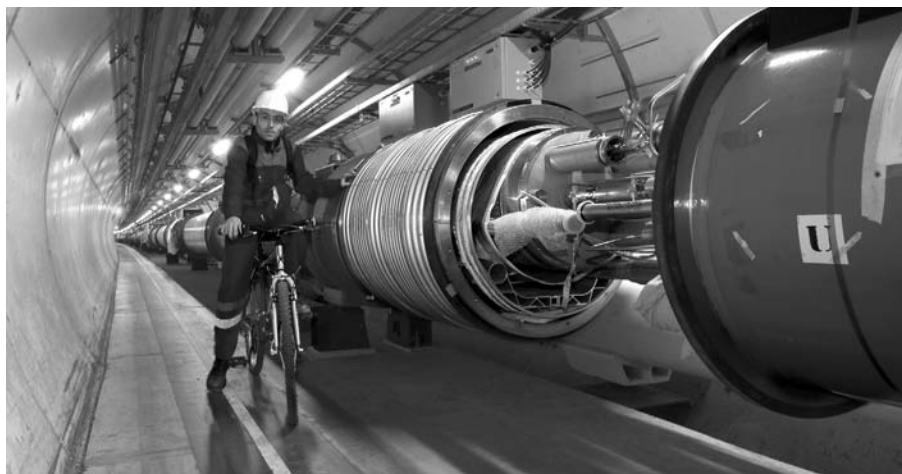
The tunnel of the Large Hadron Collider at CERN showing the beam pipe, cryogenic piping, and a few of the 9300 superconducting magnets that encircle the 27 km accelerator ring. The same bending and focusing magnets can be used for positively or negatively charged particles moving in opposite directions. Technicians move through the long tunnel on bicycles and electric carts. The LHC, the largest machine in the world, began scientific operations in 2010. [CERN.]
